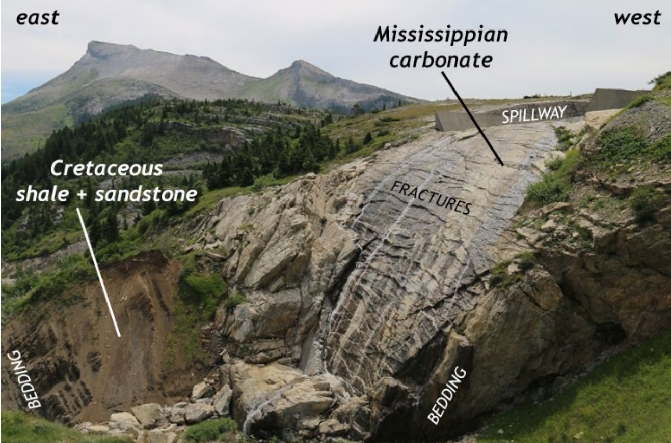
Swift Dam's spillway showcases a 3D view of the contact between folded Mississippian carbonate and Cretaceous siliciclastic strata. This is the steep, short, eastern limb of the fold. Callan Bentley photo
